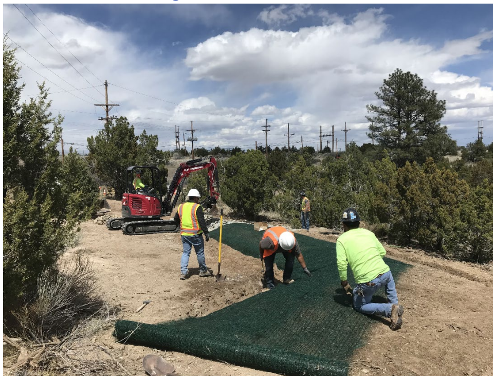
Earthen berm construction at CHQ-SMA-1.02
