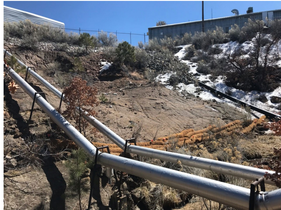
Soil removal area at SWMU 03-056(c) with existing stormwater controls.
