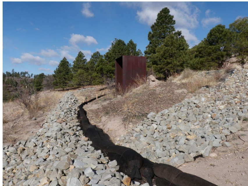
New stormwater controls at PJ-SMA-11
